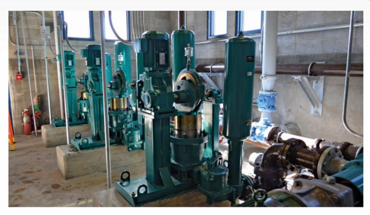
Model PE-9-SS Plunger pump in a Riverside County, California wastewater treatment plant. The facility replaced rotary lobe pumps with next generation plunger pump technology. The space saving design shown reduces the pump footprint by 35%. Application involves pumping thickened fermented sludge from a digester.
