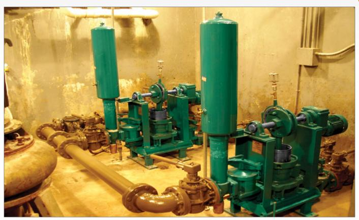
Space Saver's transferring sewage at a Knoxville, Tennessee sanitary district plant. With no base requirements, your Space Saver plunger pump options are almost endless.
