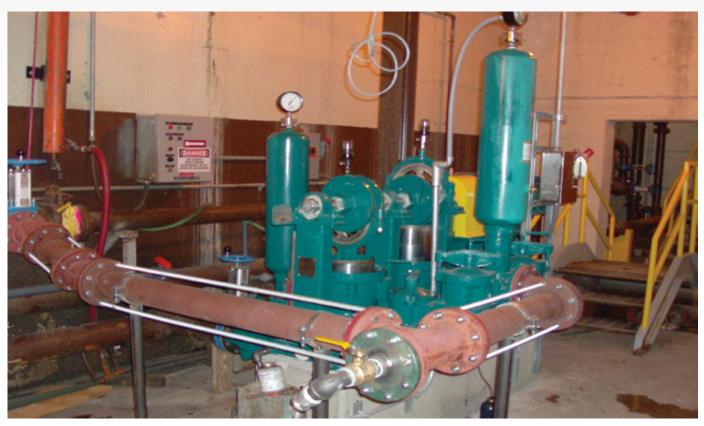
Wastecorp HPE 1142 plunger pump at an upstate New York sewage treatment facility. This facility has used plunger pumps for their primary sewage process for over 40 years. This new pump is a direct replacement.
