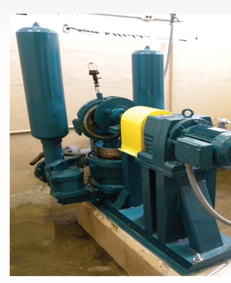
Wastecorp PE-941 Series at a Palm Beach County, Florida wastewater treatment plant. The PE-941 Series is one of the most popular plunger pump makes to replace rotary lobe and progressive cavity pumps.
