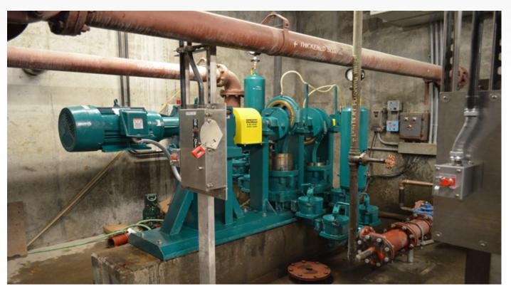
HPE-1142 plunger pump at a Boston, MA water pollution control facility. Pump includes a direct drive motor with a block heater to manage seasonal changes in weather. Higher head application which included dual ball valves for thicker slurry and sludge.
