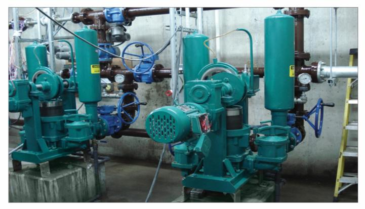
This Space Saver in Washington State replaced an existing double disc pump installation. No piping changes were needed because the pump configuration is similar.
