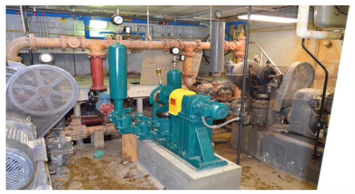
Model PE-941 dual ball valve at an upstate New York municipal sewage treatment facility. Facility upgrade involved upgrading control panels and pumping equipment. Wastecorp replaced Komline Sanderson and Carter plunger pumps. Dual ball valve configuration assists in pumping high solids above 15%.
