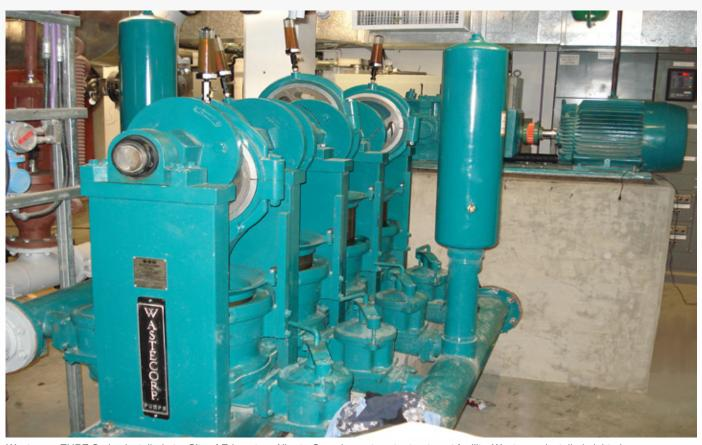
Wastecorp EHPE Series installed at a City of Edmonton, Alberta Canada wastewater treatment facility. Wastecorp installed eight plunger pumps at the facility as part of a multi-year upgrade/expansion.
