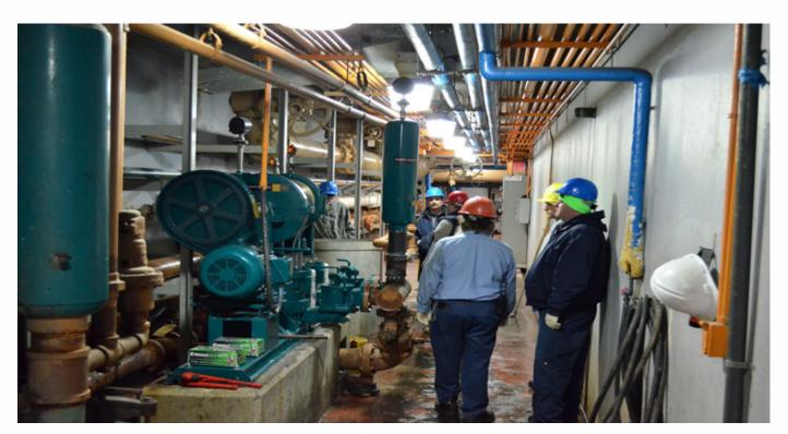
HPE 81W at a New Jersey wastewater treatment plant. The belt driven model has been favored by this facility's operators for decades. When it was time to replace the existing plunger pump the operators opted for the same belt driven design for enhanced pumping productivity.
